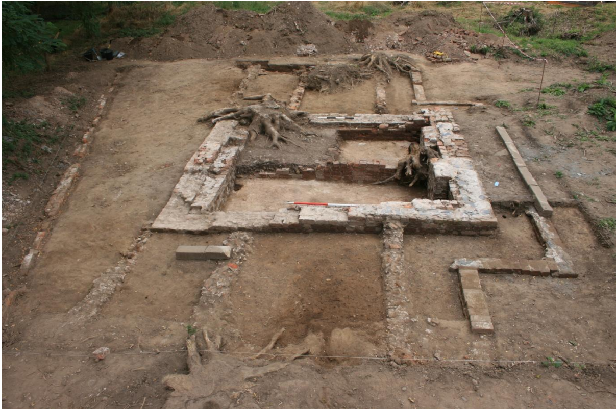
14. General view, looking west, of the building at its maximum extent with the robber trenches and surviving footings of the east wing (foreground) and the west wing (background). Note the enclosure wall 342 at a divergent angle on the left (south)
