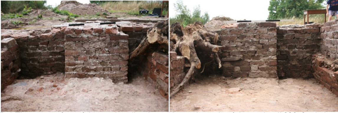
5, 6 The interior face of the north wall – shots taken either side of the axial wall 338. Single-brick joist-supporting walls 339 and 340 can be seen extreme left and extreme right
